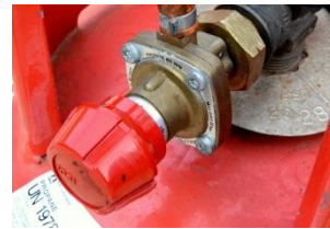
Fig 2. Regulator valve
