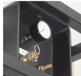
Fig.3 Pressure, fill point and pressure relief.
