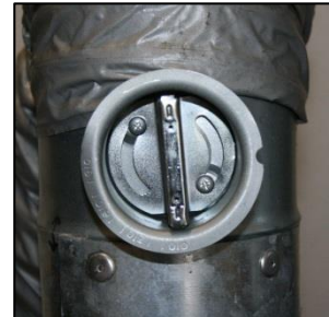
Fig 14. Fog valve fully open
