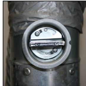
Fig 13. Fog valve fully closed
