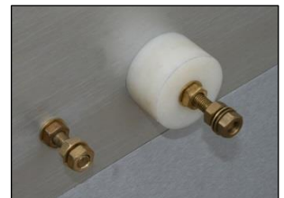
Fig 3. Wire connection points
