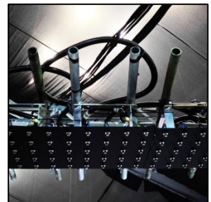
Fig 5. Scaffold pole mounting
