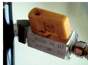
Fig.5 Yellow filling lever in 'open' position
