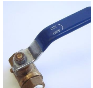
Fig 4. Bulk supply lever in 'off' position
